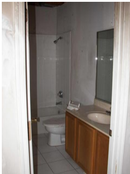
Fire damaged metal framing in the laundry room
